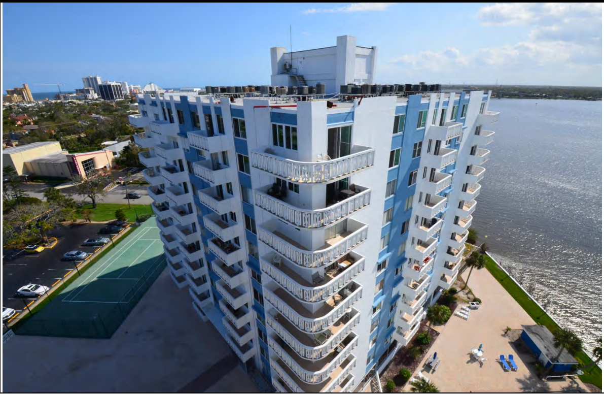
EXTERIOR VIEW OF SOUTH TOWER BUILDING
