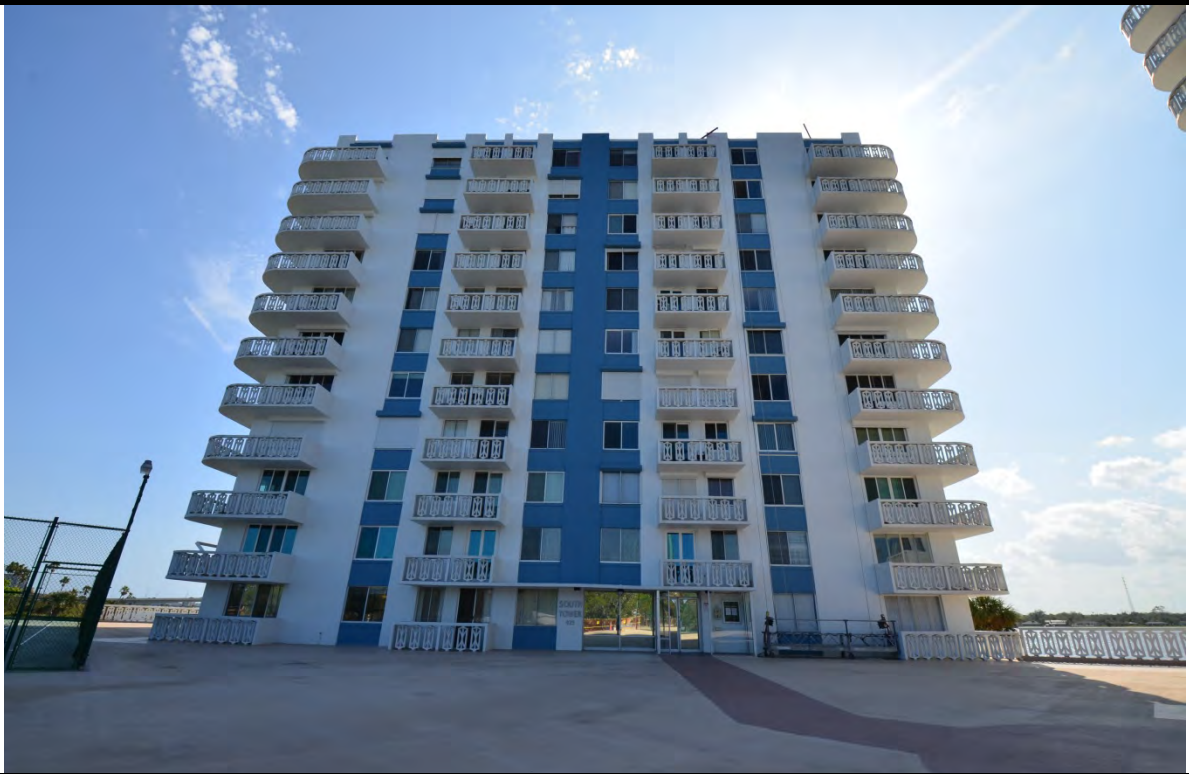
EXTERIOR VIEW OF SOUTH TOWER BUILDING
