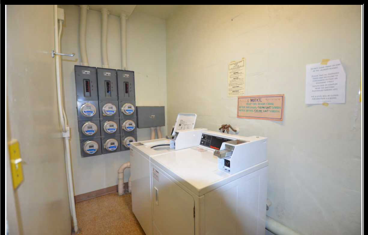
INTERIOR VIEW OF TYPICAL COMMON AREAS
