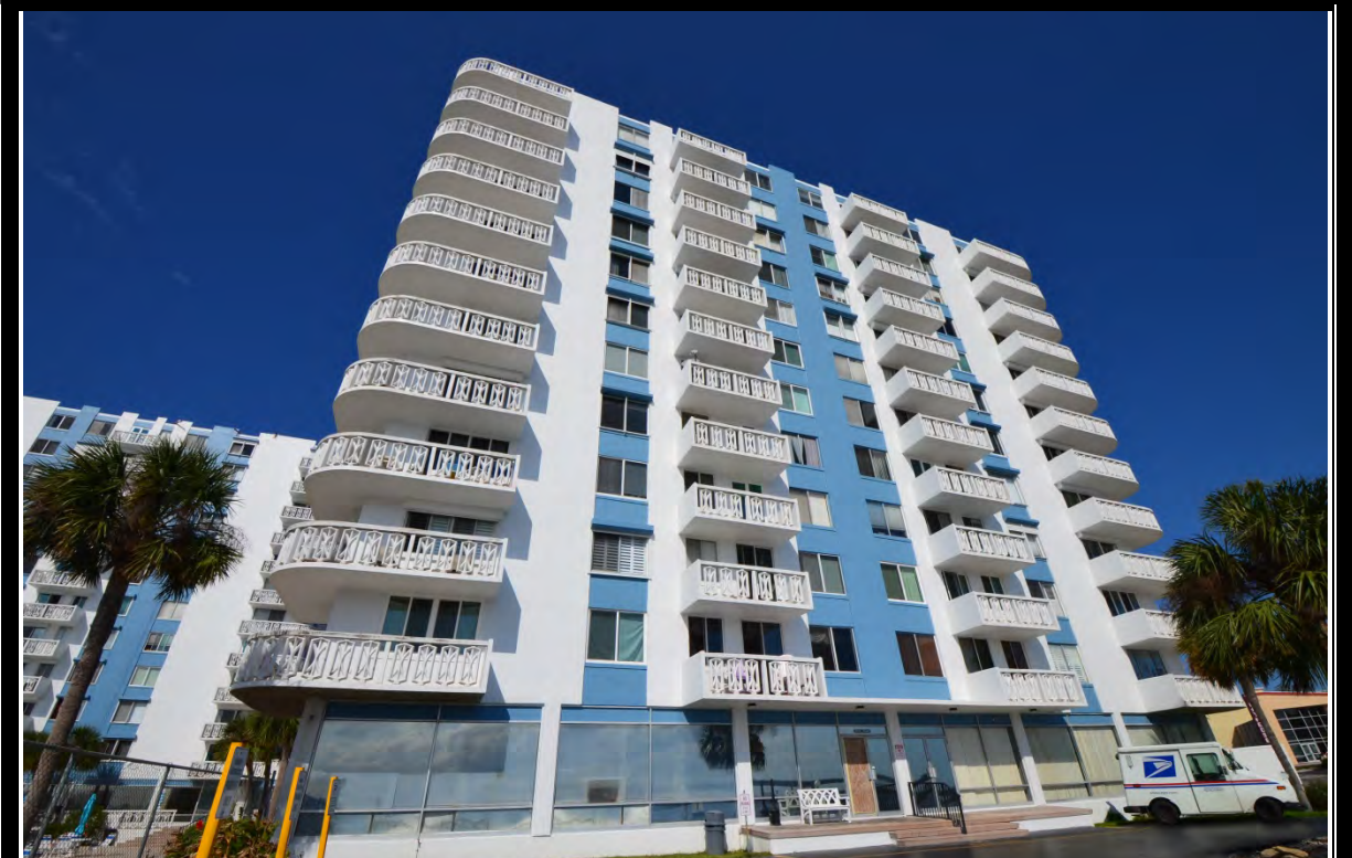
EXTERIOR VIEW OF SOUTH TOWER BUILDING
