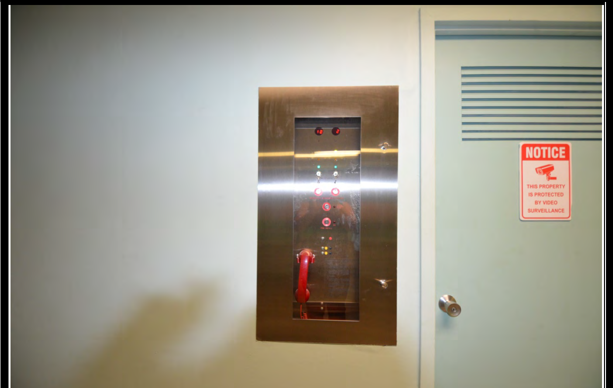
VIEW OF TYPICAL BUILDING MECHANICAL EQUIPMENT
