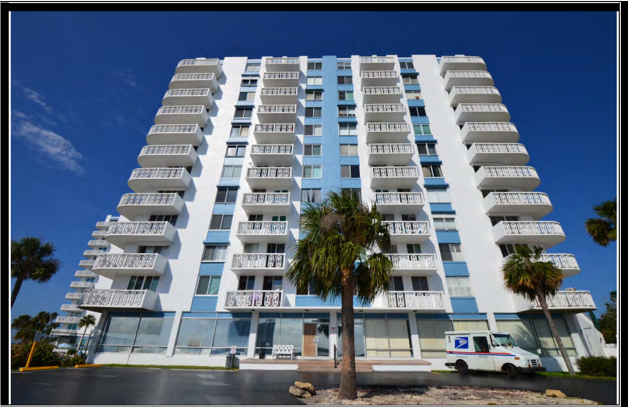
EXTERIOR VIEW OF SOUTH TOWER BUILDING
