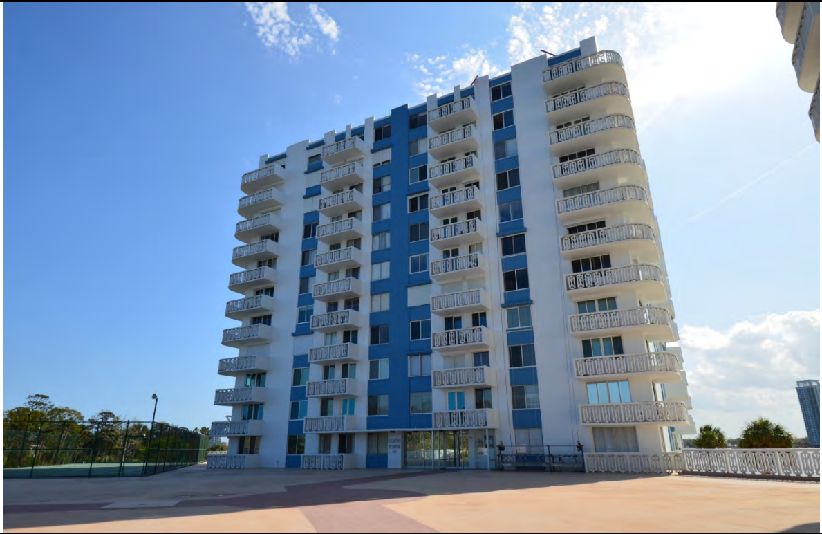
EXTERIOR VIEW OF SOUTH TOWER BUILDING
