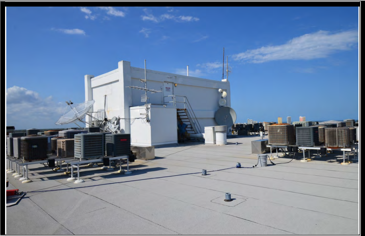
VIEW OF ROOF
