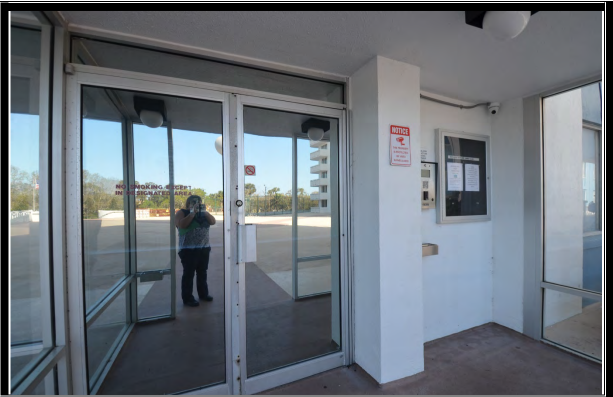
EXTERIOR VIEW OF SOUTH TOWER BUILDING
