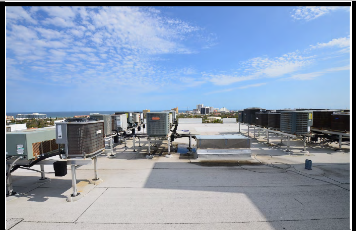
VIEW OF ROOF
