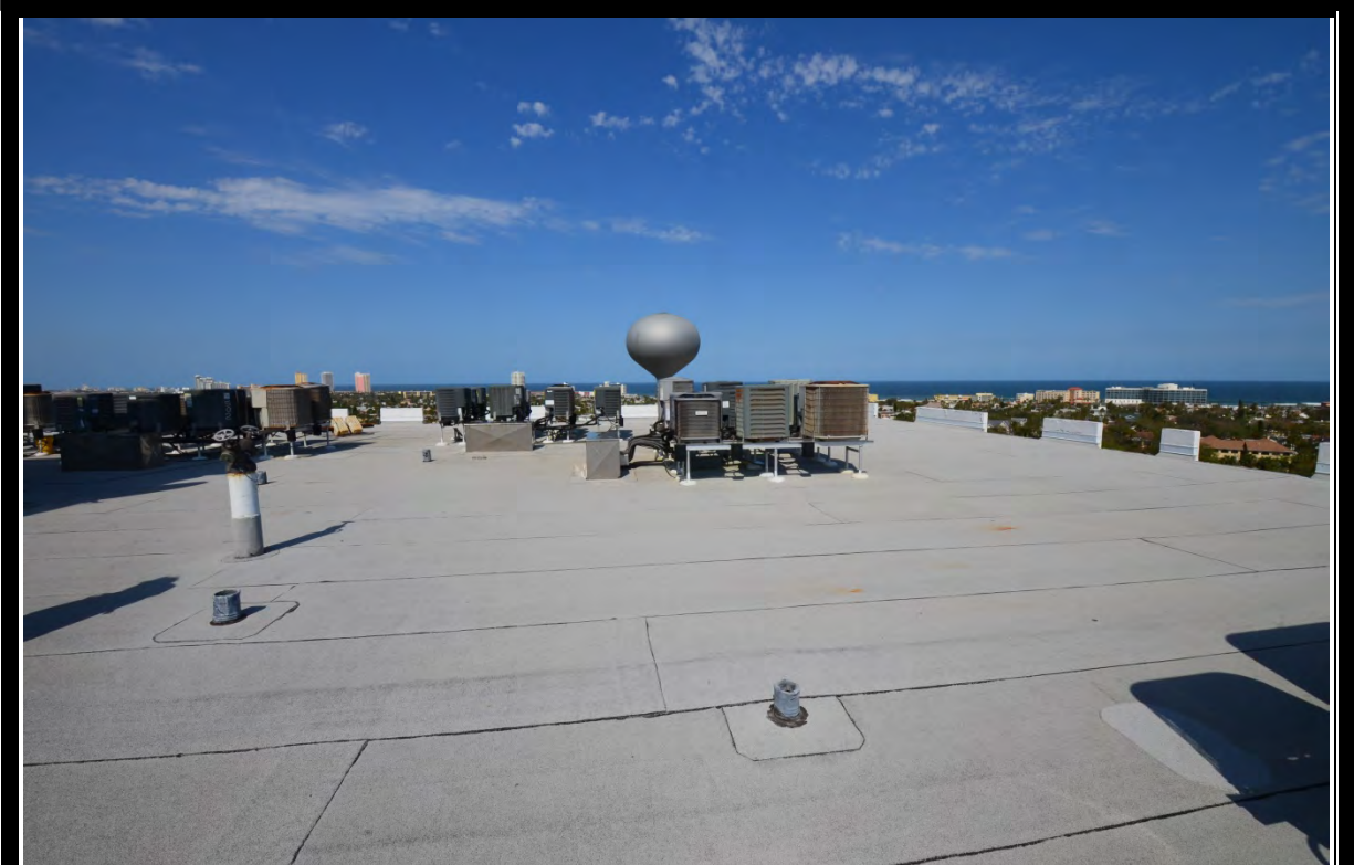
VIEW OF ROOF
