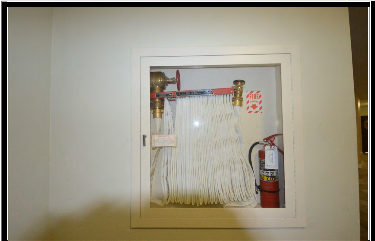
VIEW OF TYPICAL BUILDING MECHANICAL EQUIPMENT
