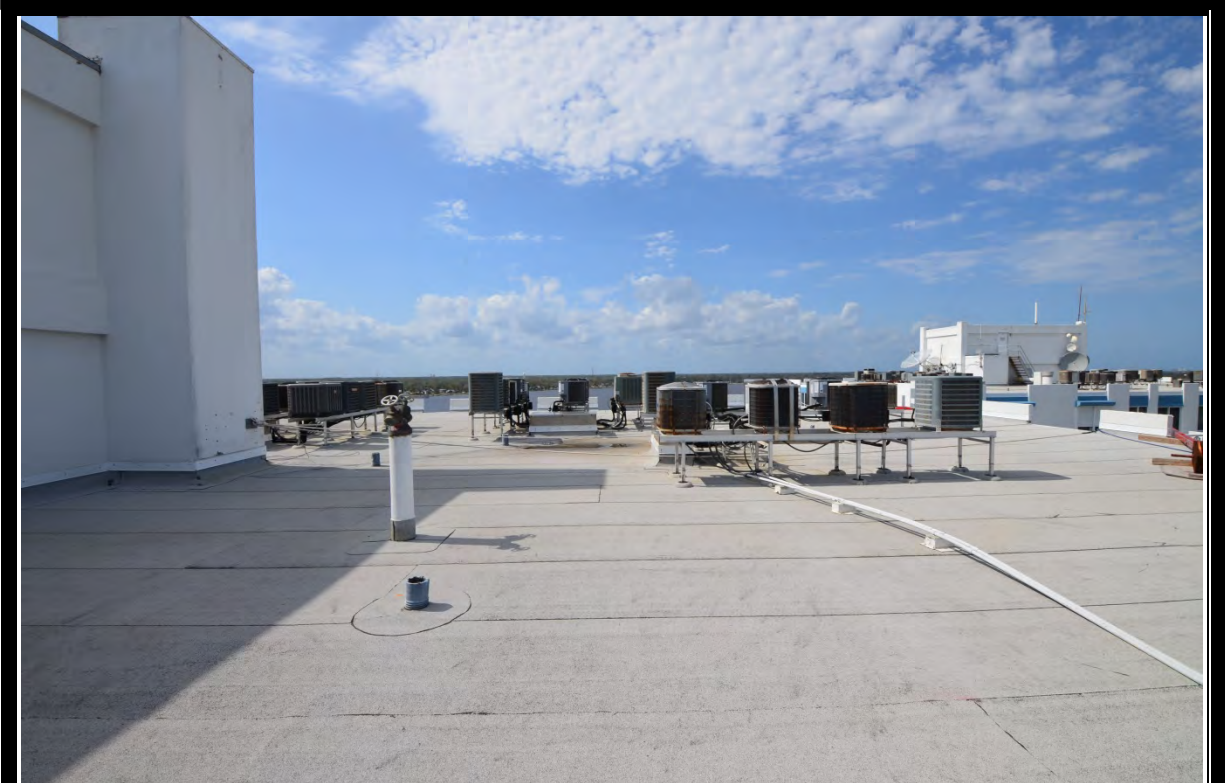
VIEW OF ROOF
