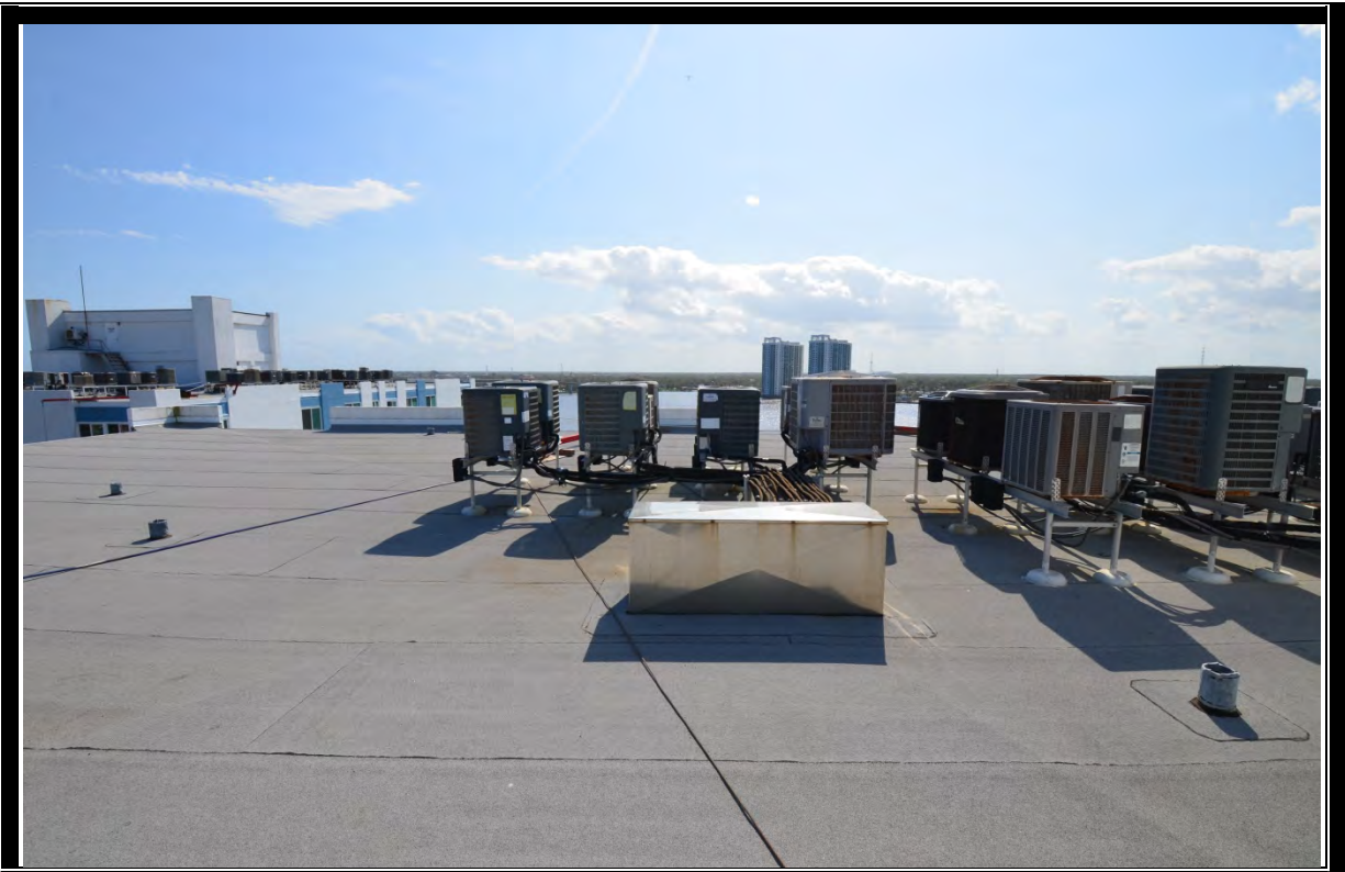
VIEW OF ROOF
