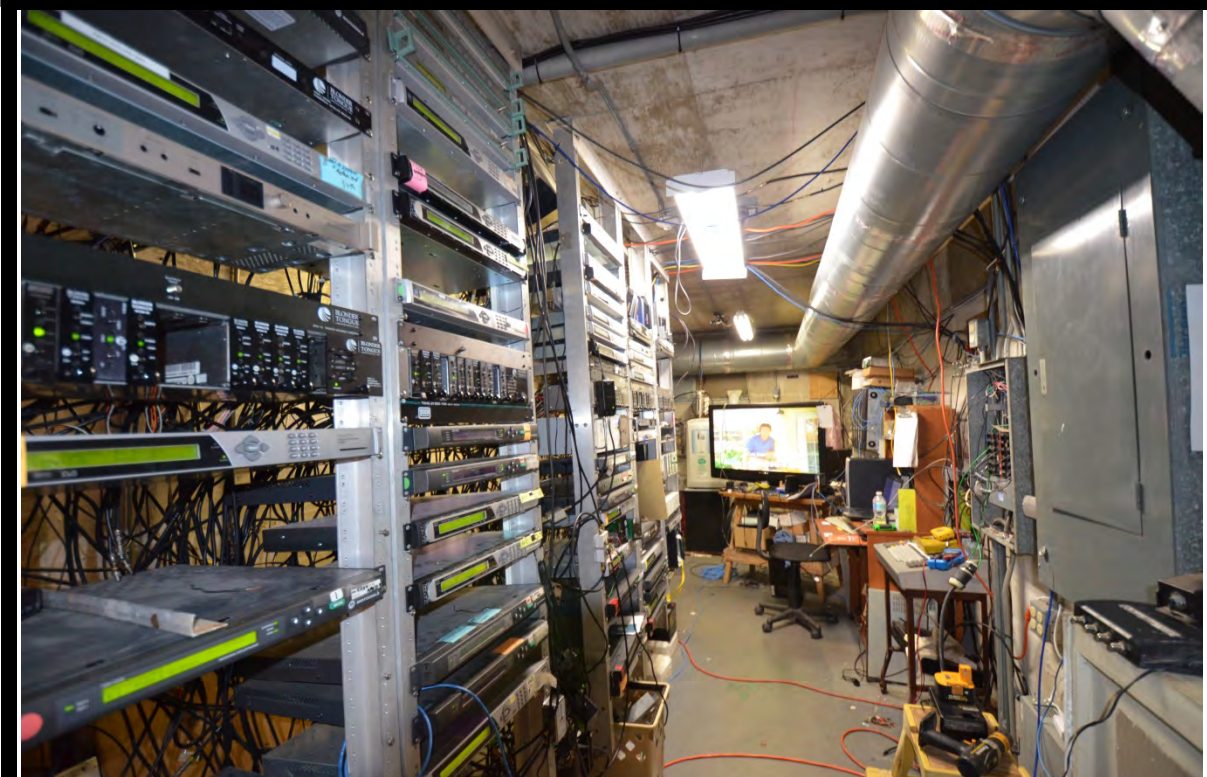
VIEW OF TYPICAL BUILDING MECHANICAL EQUIPMENT
