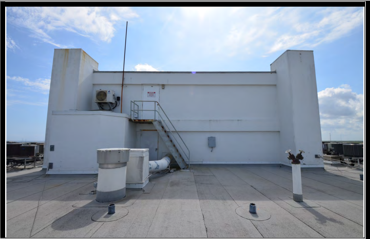
VIEW OF ROOF
