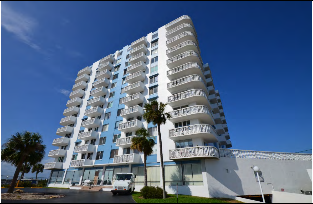
EXTERIOR VIEW OF SOUTH TOWER BUILDING
