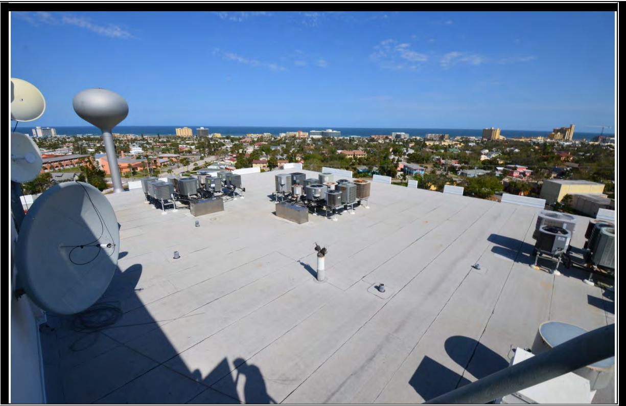
VIEW OF ROOF
