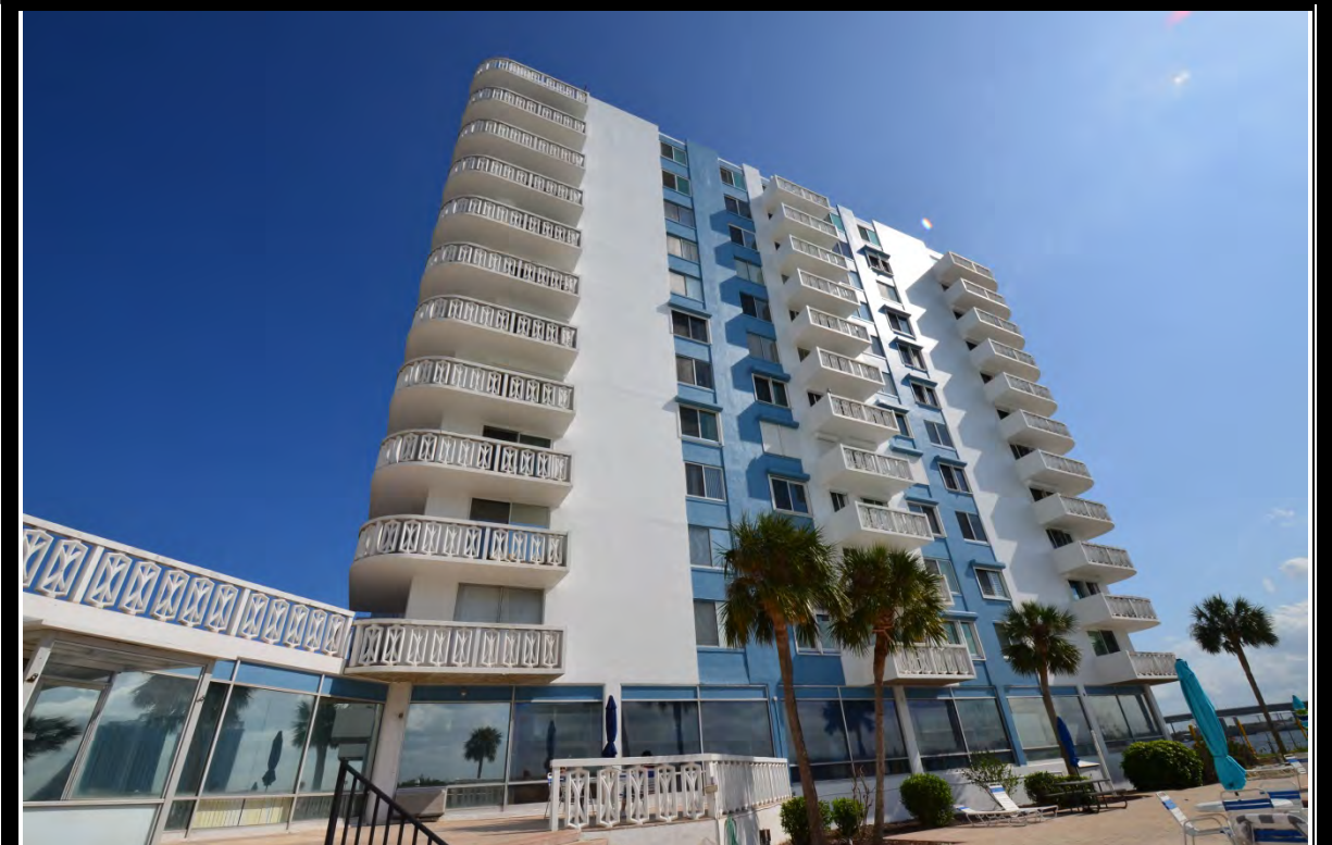
EXTERIOR VIEW OF SOUTH TOWER BUILDING
