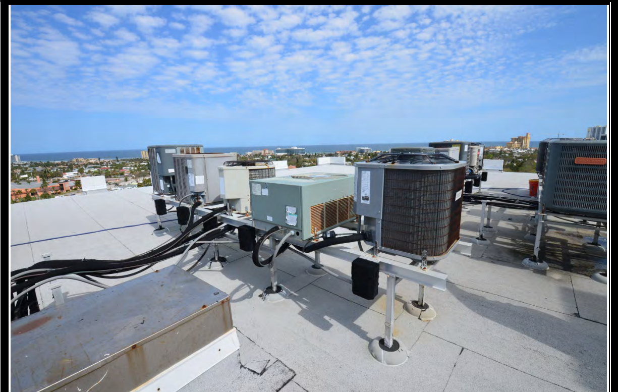
VIEW OF ROOF
