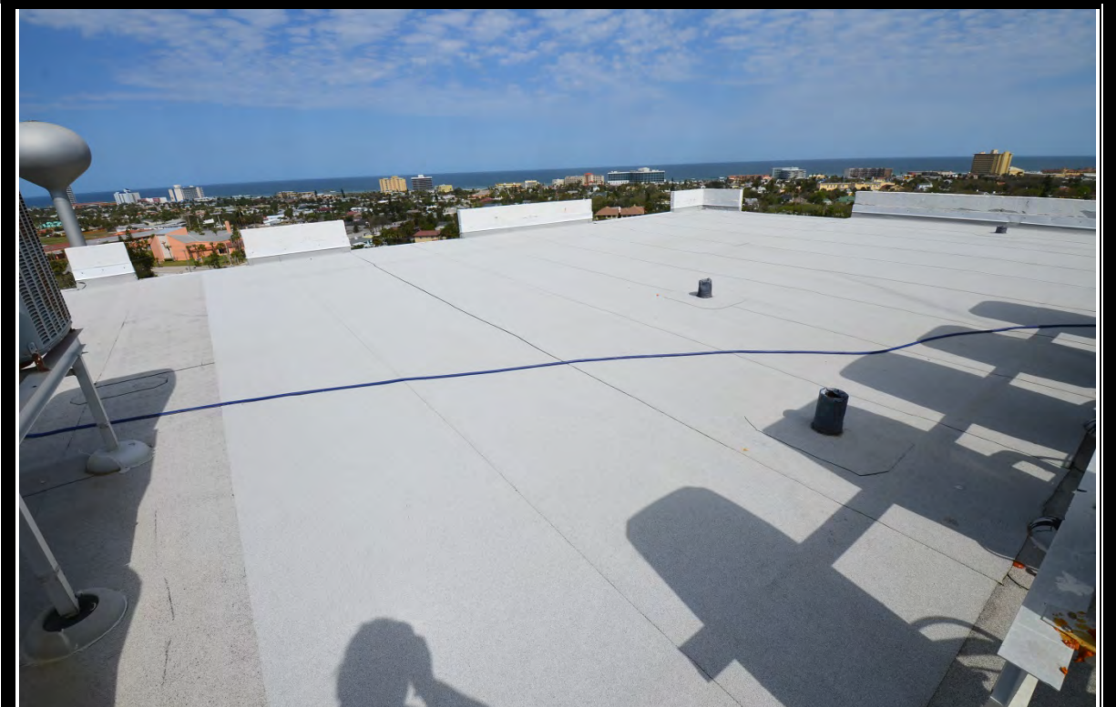
VIEW OF ROOF
