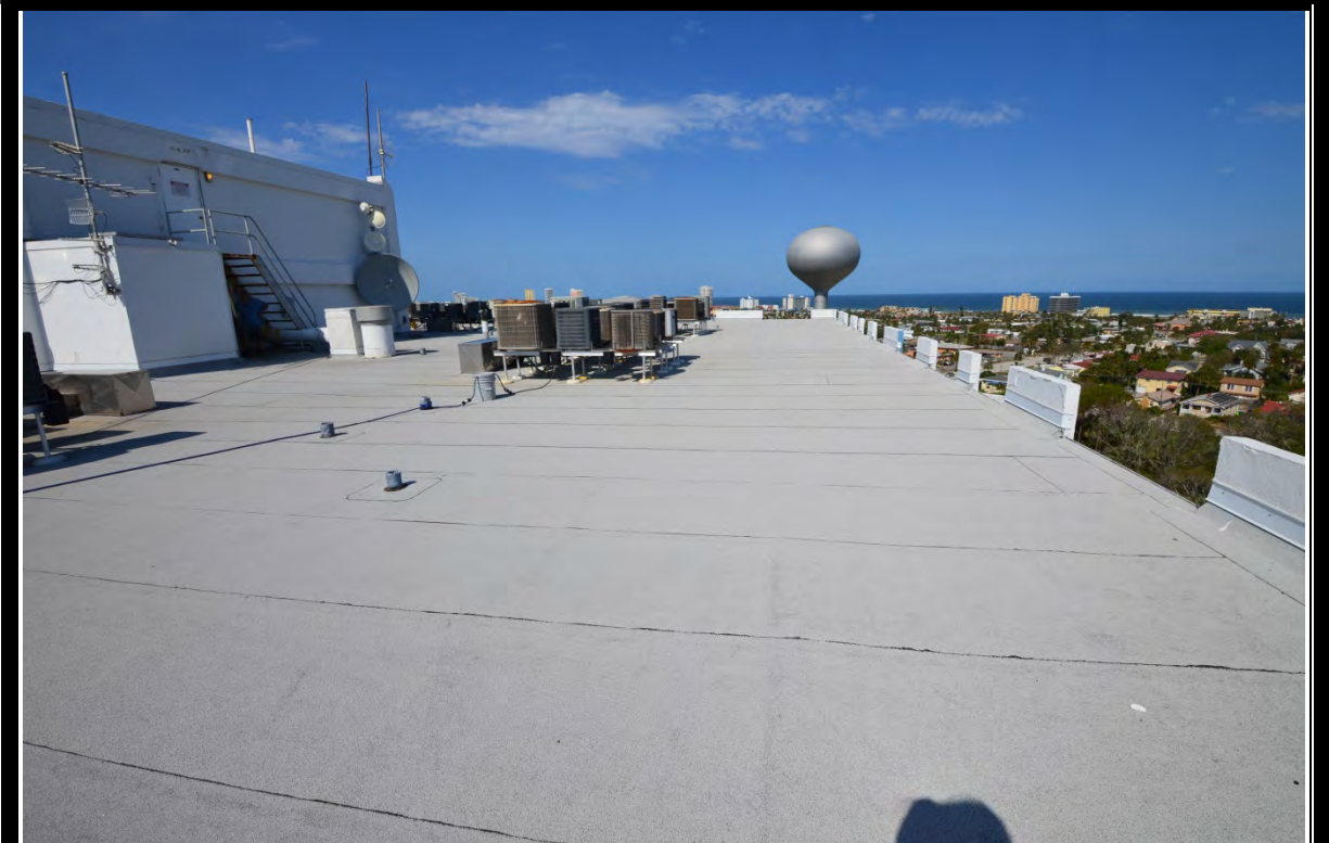
VIEW OF ROOF
