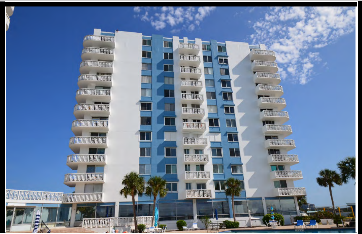
EXTERIOR VIEW OF SOUTH TOWER BUILDING
