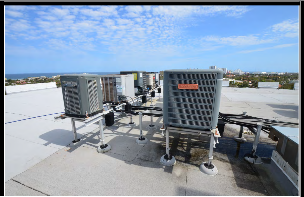
VIEW OF ROOF
